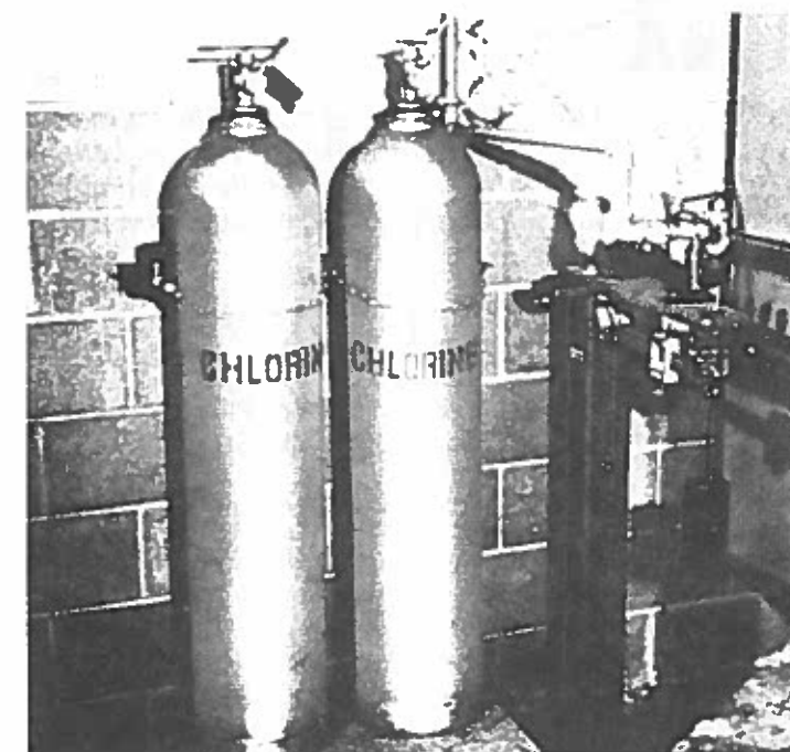
Fig. 5.17 Typical chlorine cylinder station for water treatment (Courtesy of PPG Industries)
